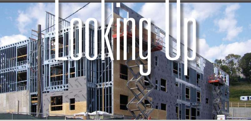
Each piece of cold-formed steel was ordered cut to length, including the 6-inch wall studs, by Marino\WARE, South Plainfield, N.J.
